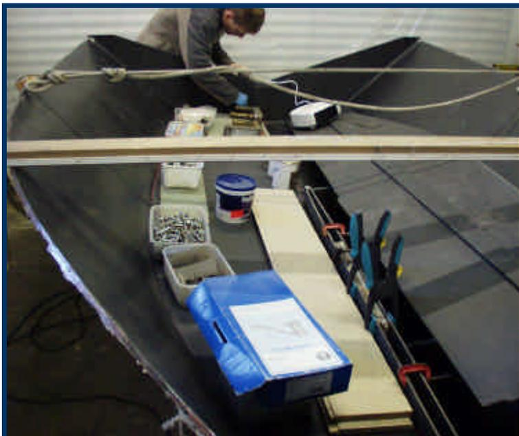
Photo 15 (right) shows the floor after the joints have been taped
