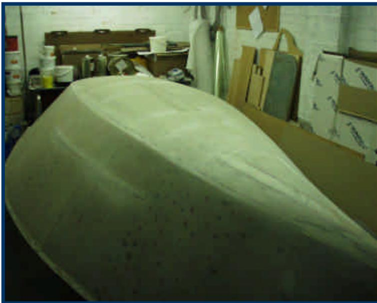
Photo 3 (above) shows hull foam after smoothing. Take care when fairing around any epoxy hard spots (around the pin holes) as the foam will sand more easily than the epoxy and you can end up with low spots
